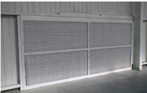
FLUSH WALL MOUNTED MASTERFLO FILTER WALL
