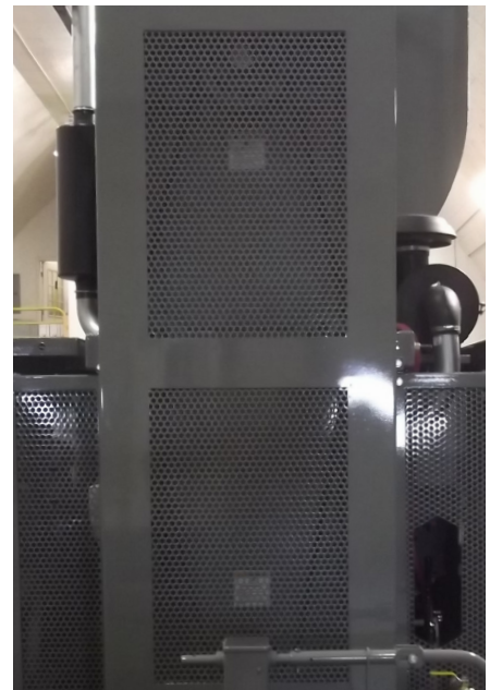
Figure 31: Fan drive belt guard
