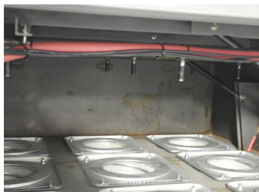
Figure 33: Pulse system inside filter bay
